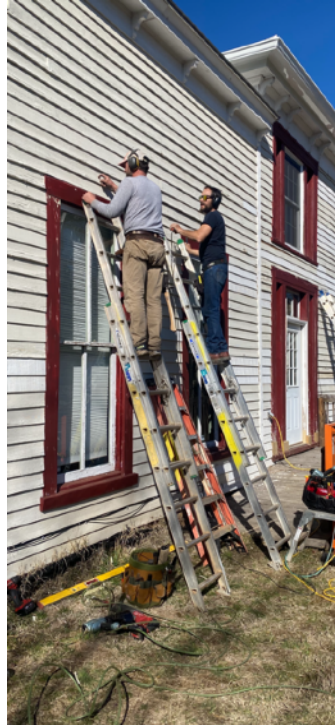
Repairing and replacing siding at the Graffiti House in February 2024
