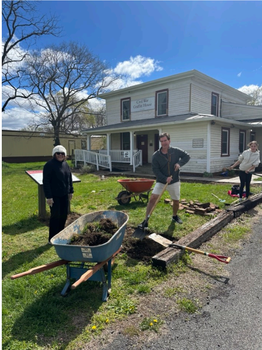
Park Day at the Graffiti House in 2024; Brick walkway work.
